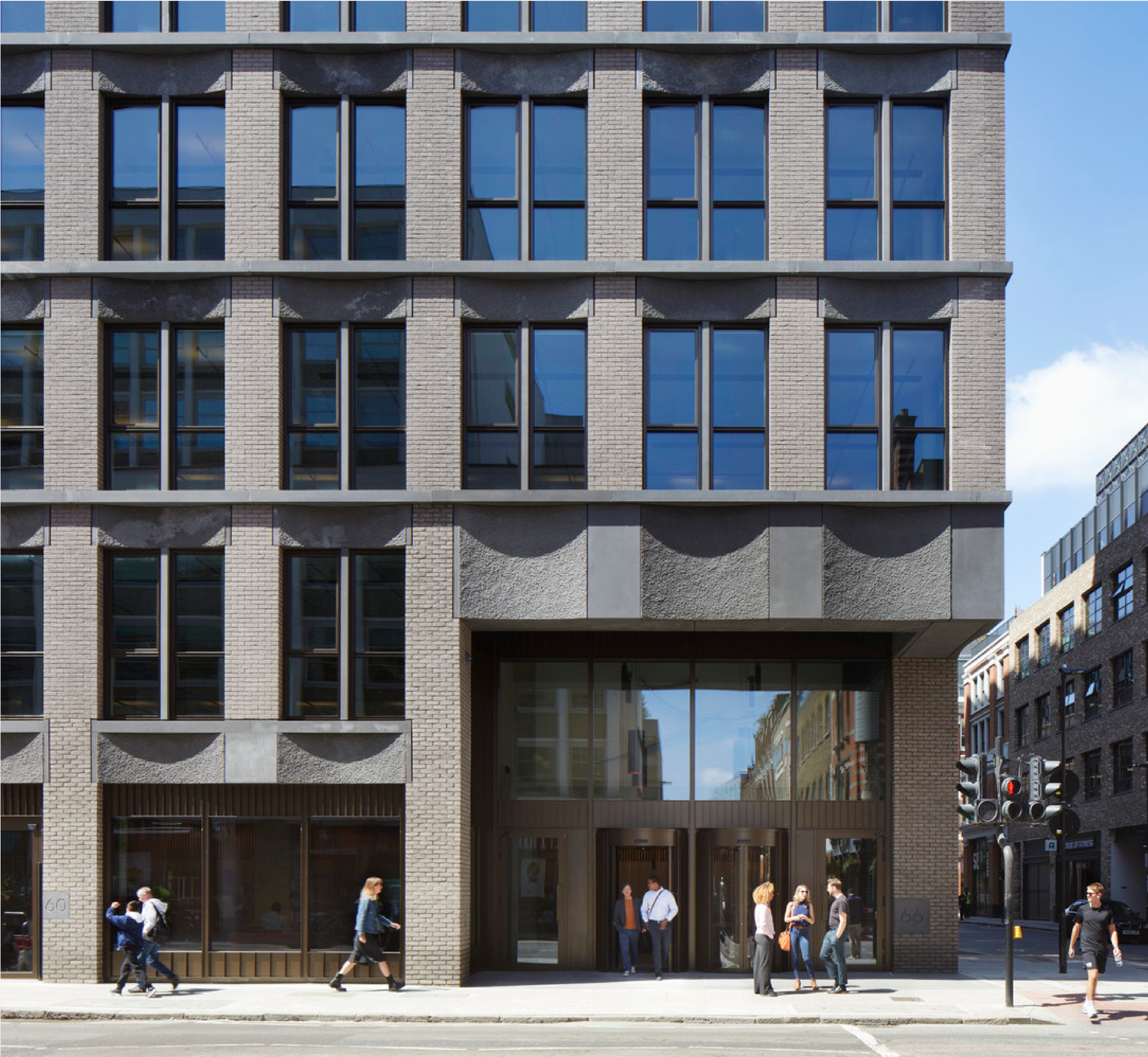
Sixty Six City Road, Old Street ECI
